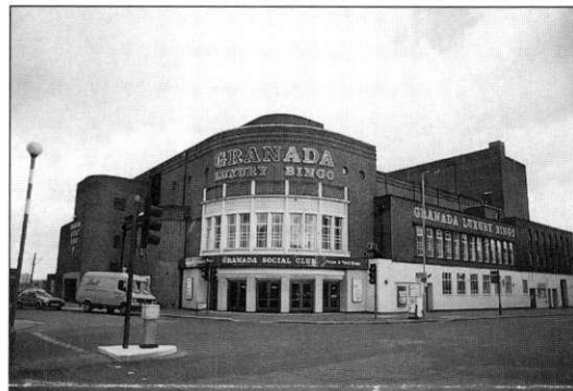
Clapham Junction Granada: exterior
