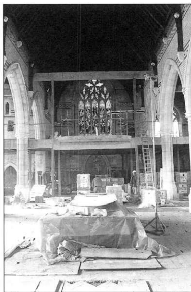
Work in progress on the alterations to St Barnabas' Church
