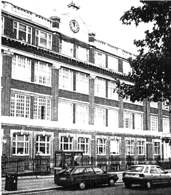
George West House in 1998 before refurbishment
